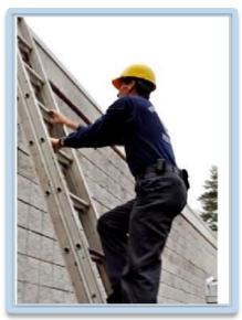
In the photo above, the worker is safe because the base of that 20 foot ladder is 4 feet (or ¼ of the working height) away from the 16 foot wall.
